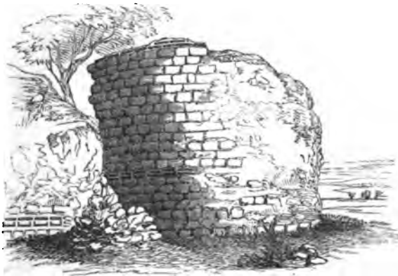
External view of a tower on the western side.
